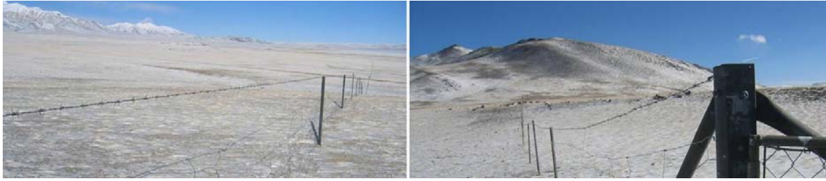
Figure 7. Fencing constructed in 2006 across parts of the Aru Basin, the left photo showing the division between Gertse and Rutok Counties, and the right photo a livestock enclosure to promote the “return of pasture to grassland” but located within an antelope migration staging area in the southern basin.
